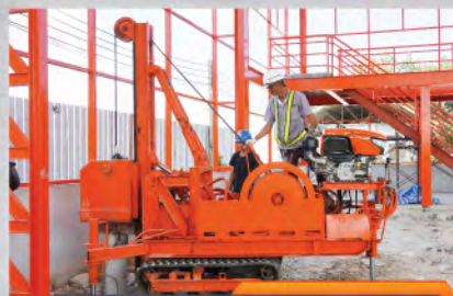
Micropile installation Suitability of horsepower 12.5 - 15.5 HP
